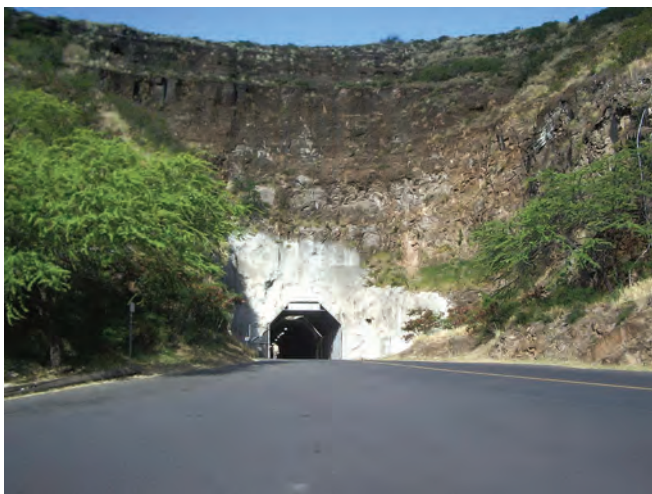
Tunnel into the volcano crater at Diamond Head. The tunnel entrance has gates to seal the crater and a cover to catch falling rocks
